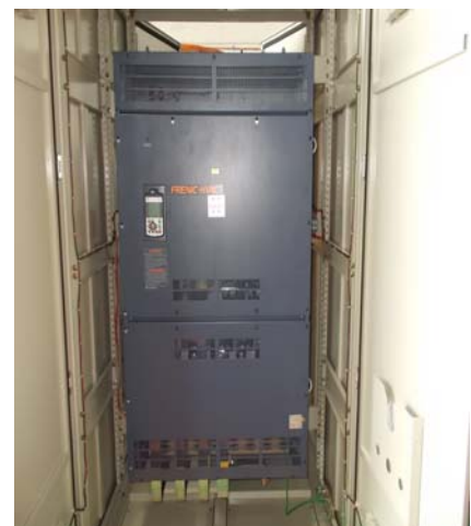
Figure 8.0C VFD Starter Cabinet (Optional)
